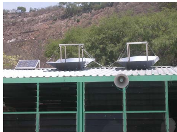
Fig. 6: Two bifacial solar panels at rural school
